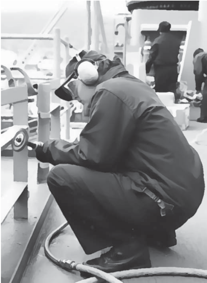
Figure 16.23 Sailor grinding a handrail
