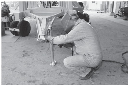
Figure B.10 After: Simple trailer jack lifts work piece and improves posture at Fleet Readiness Center East (Photos adapted from Ergonomics Guide for Welders, unpublished Navy Occupational Safety and Health Working Group, Ergonomics Task Action Team with technical support provided by the Certified Professional Ergonomists at General Dynamics Information Technology (GDIT), San Diego, CA, 2010)
