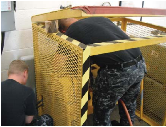
Figure 16.7 Checking connection to test equipment (Graphic by Lee Ostrom)
