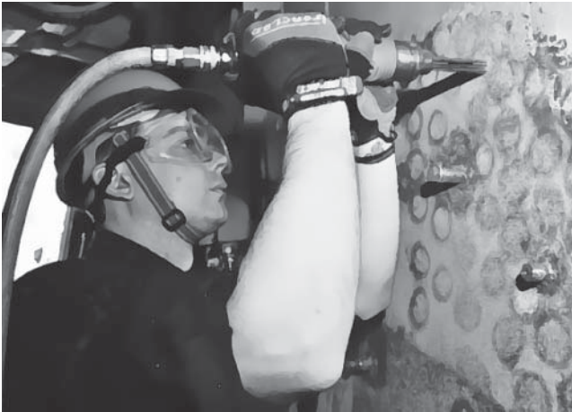
Figure 16.25 Operations specialist wears certifie antivibration gloves while using a needle gun to chip paint off a bulkhead
