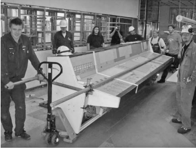
FIGURE 8.7 Old control panels are removed from the Mälarenergi control room.
