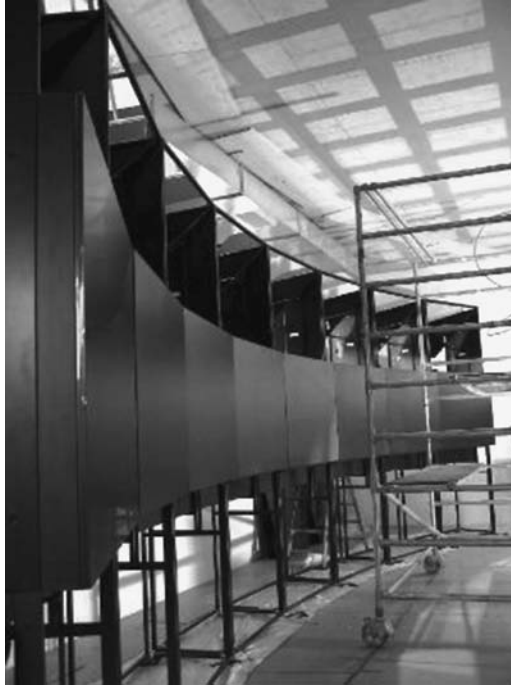
FIGURE 4.23 Large screen cube wall installed in a curved arrangement. (See colour insert.)
