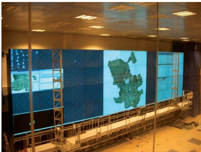
FIGURE 4.24 Installation of a very large DLP cube wall.
