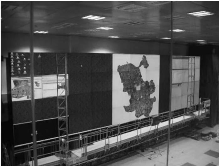
FIGURE 4.24 Installation of a very large DLP cube wall. (See colour insert.)
