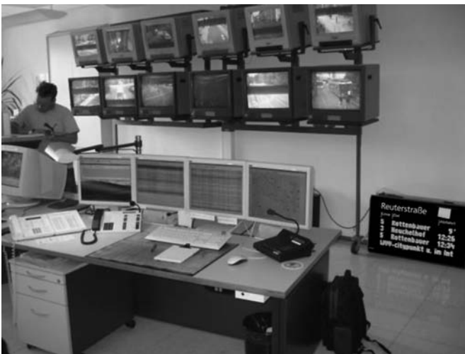
FIGURE 4.15 Example of a CRT monitor wall.
