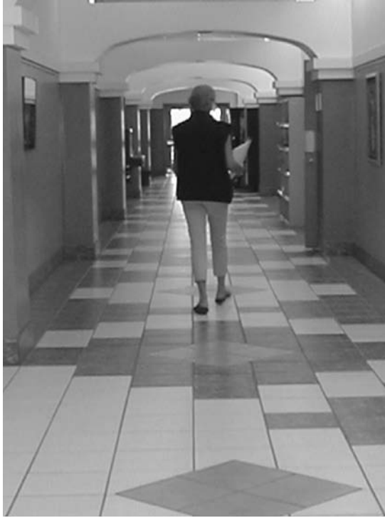
FIGURE 4.4 Complex floor patterns can confuse older adults with low vision. (Photo taken by Liu, L., 2005.)
