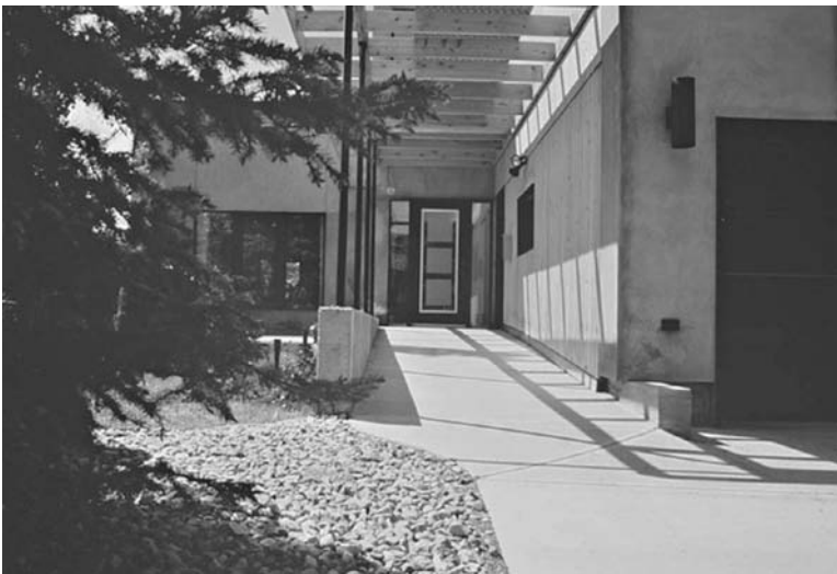
FIGURE 4.7 Front entrance of home of Ron Wickman, architect. The entrance was created to make R. Wickman’s home visitable for his father, Percy Wickman, who used a wheelchair. Percy Wickman served as a politician and was an advocate for persons with disabilities. (Photo taken by Wickman, R., 2006.)
