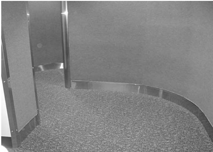
FIGURE 4.2 Door-free entrance to washroom facilitates use by people who have mobility aids and travelers with luggage. (Photo taken by Liu, L., 2004.)
