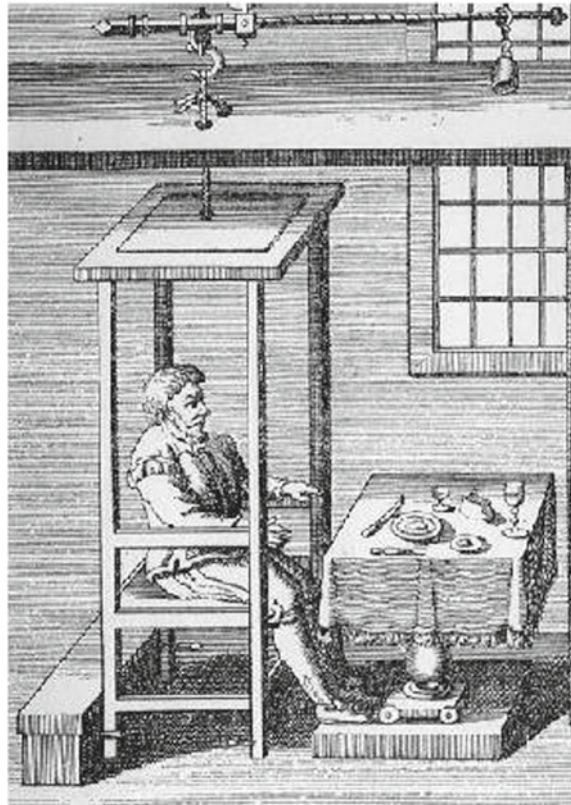
Fig. 10.1 In the seventeenth century Paduan physician Santorio Sanctorius (1561–1636), spent many years eating, sleeping and working in a ‘statical’ chair connected to the arm of a calibrated scale. He paved the way for the contemporary discipline of metabolism. (Reproduced from Heymsfield (2008). With permission)
