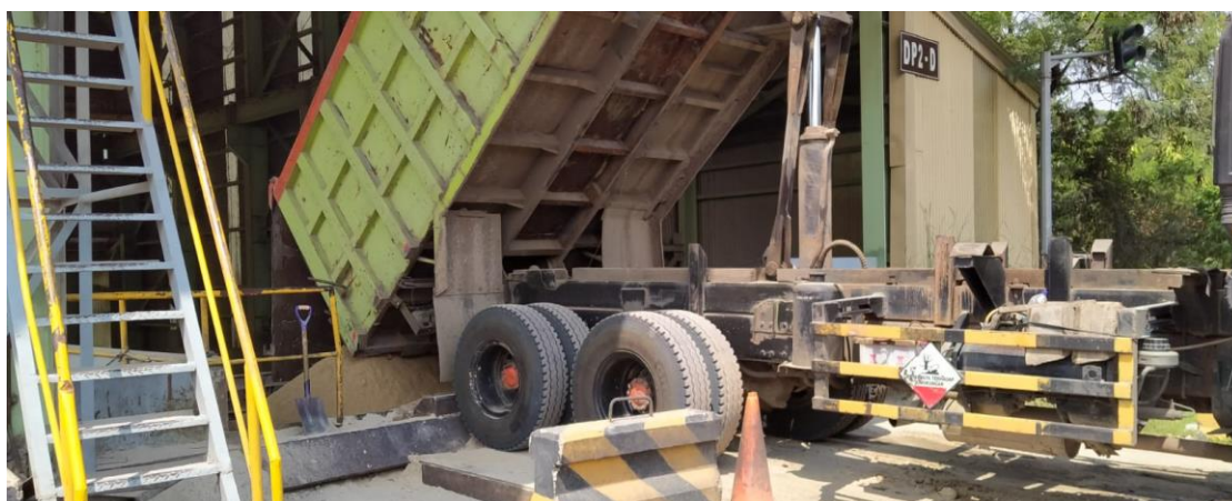
Gambar 16. Proses Unloading Material Trass
